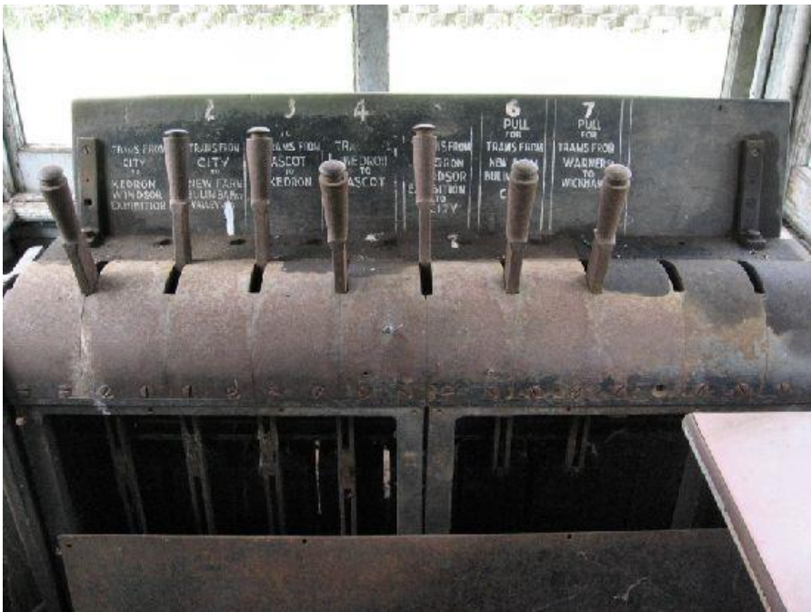
The lever frame in the Valley Signal cabin now at the museum.
