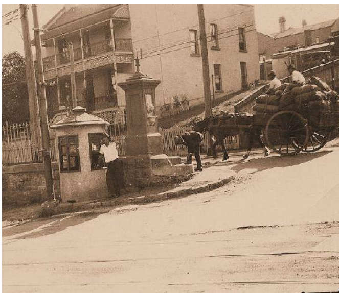
Left :- The points Cabin that was in Countess St.
