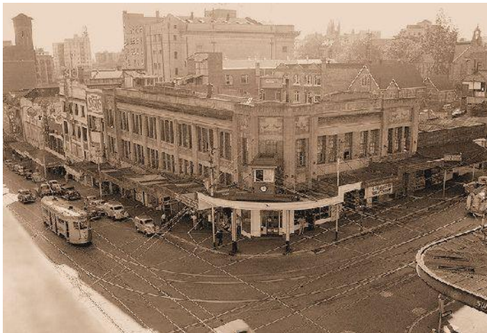
Left:- The Wharf Street Signal Box. The building behind the box was known as Adelaide House and was demolished to build the Taxation Building.
